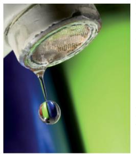
Figure 11Build-up of limescale on an aeratingtap outlet.
